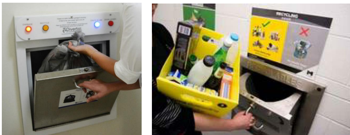
Figure 5-4 Example chute disposal access points
